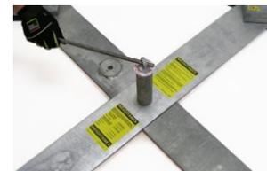
Using the supplied Tommy bar Hand tighten the eyebolt firmly in place until it is fully located..
